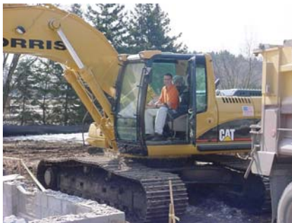
Shaun puts the finishing touches on demolition
